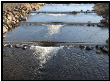
New notched cross-channel vanes on Mill Creek
